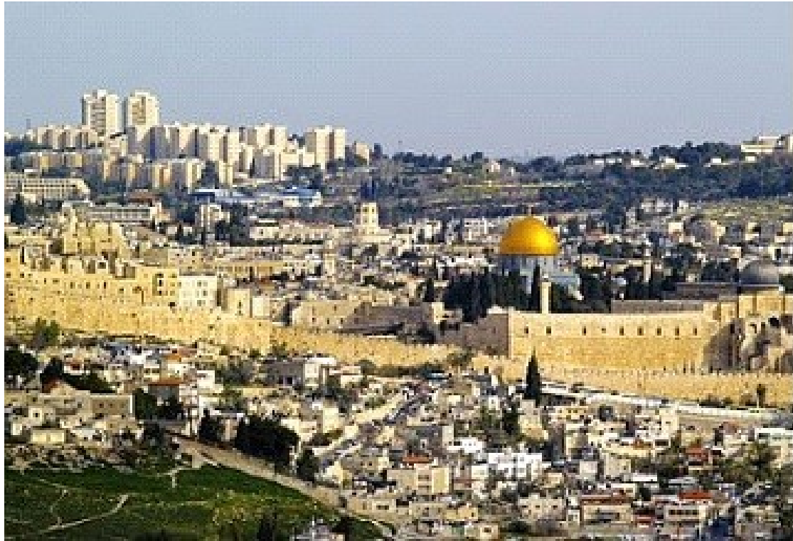
Figure 01.16. Since ancient times, the city of Jerusalem has been surrounded by walls.
